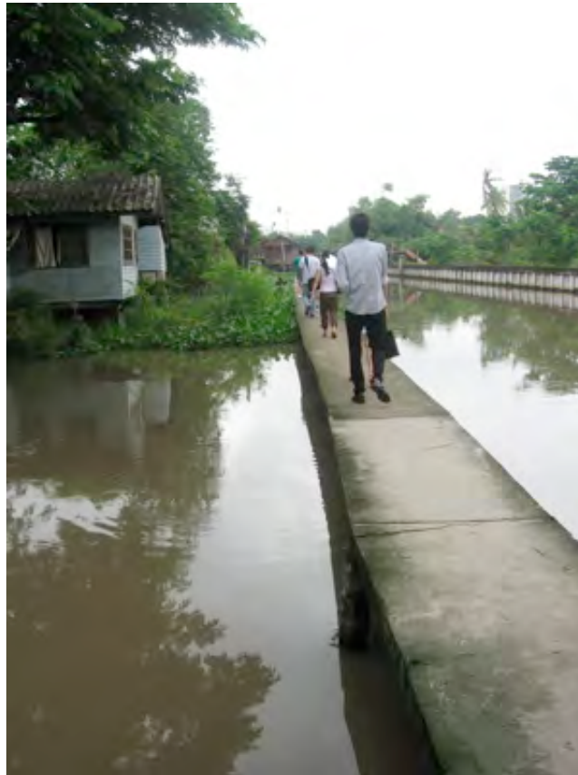
Concrete walkway along a canal
